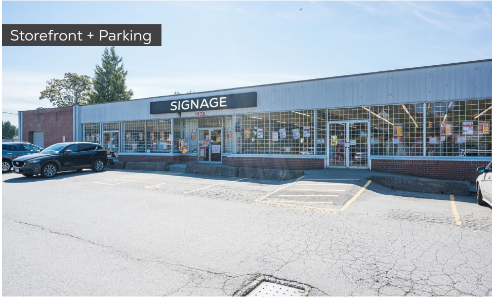
Main Entrance off SE Marine Dr
