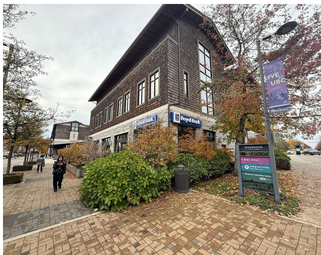
Corner Berton Ave and Wesbrook Mall
