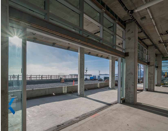
Aire West - Unit 1, Covered Patio, Looking West
