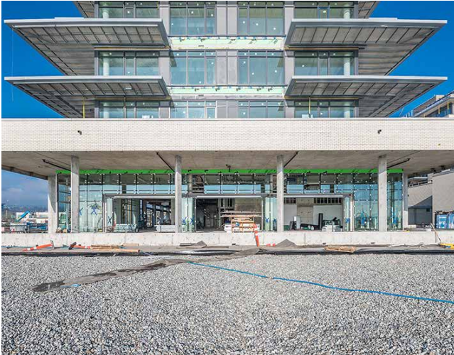
Aire West - Restaurant Unit, Front View
