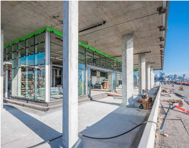
Aire West - Unit 1, Covered Patio, Looking East
